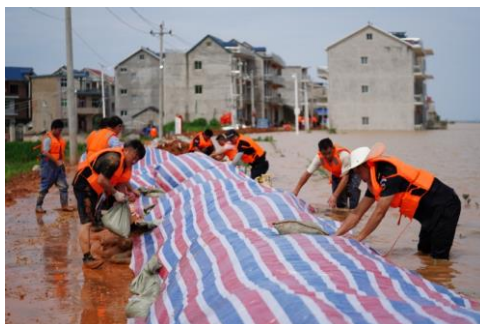
A flood barrier is reinforced with waterproof material.
